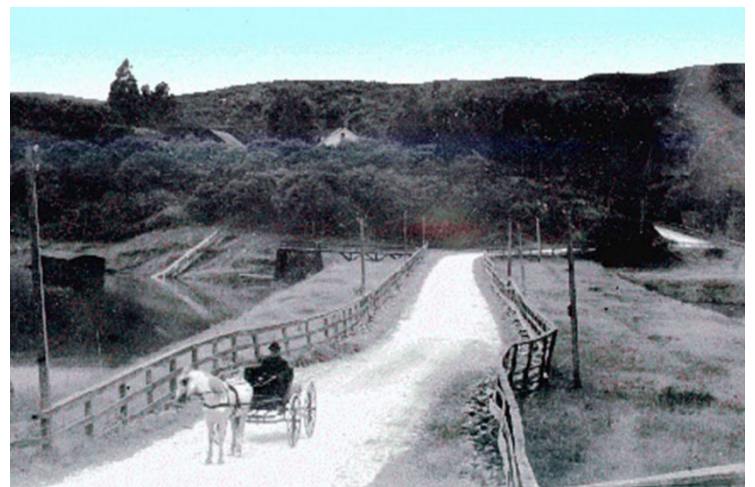
Bridge over Crystal Springs Reservoir showing the shift in the ground following the earthquake. The San Andreas Fault runs down the middle of the reservoir. –Courtesy USGS
