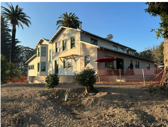
Rebuilt Steele house at Pie Ranch --Photos courtesy of Jered Larson
