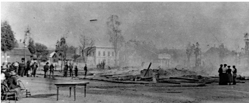
The Levy Brothers Store before and after the earthquake –Half Moon Bay History Association
