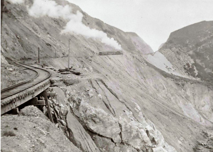
Showing the Ocean Shore Railroad on the section of San Pedro Mountain where much of the hillside had slid into the ocean only a few years earlier –Half Moon Bay History Association
