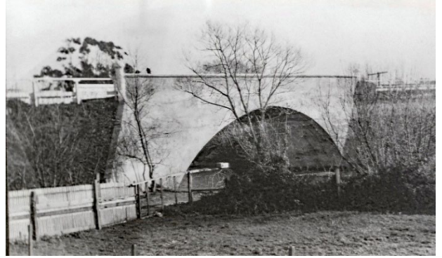
Main Street Bridge over Pilarcitos Creek –Half Moon Bay History Association
