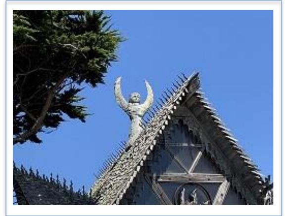
The A-frame is built in the style of a Norwegian stave church—using poles or “staves” —and was constructed starting in 1973 using long eucalyptus trunks harvested from the hills above El Granada. The main timbers in the A-frame are from an old water tower that once stood next to Cabrillo Highway.
