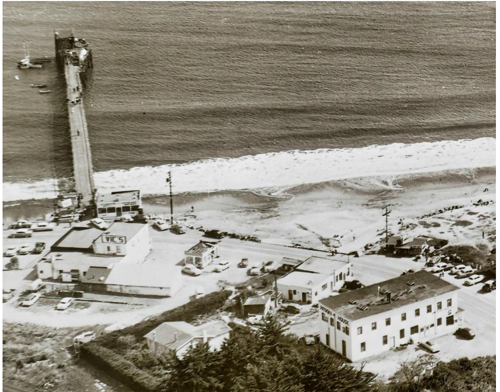
Patroni's Wharf in the upper left and the Patroni House in the lower right
